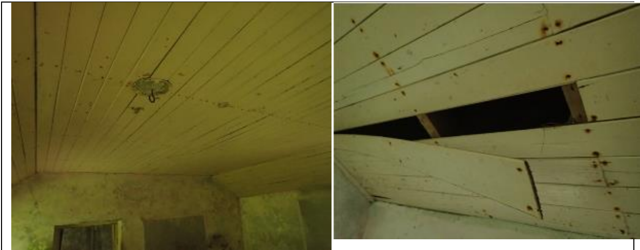
Timber lat ceiling
